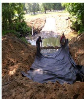
*This stream crossings construction, when finished, will allow animals to cross without eroding the soil or destroying the steambanks*
